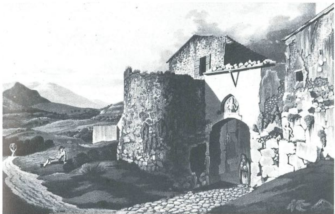
EXTERIOR VIEW OF THE PORTA SAN PIERO AT ALATRI.
